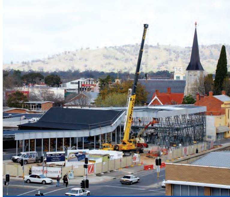
Under construction: Albury City’s new Library Museum, at the forefront of the trend in cultural facilities convergence
